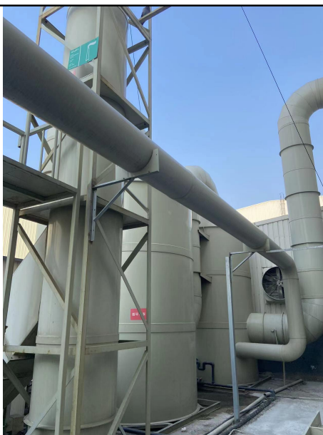
喷漆废气处理设施：喷淋塔+UV+二级活性炭，DA006
