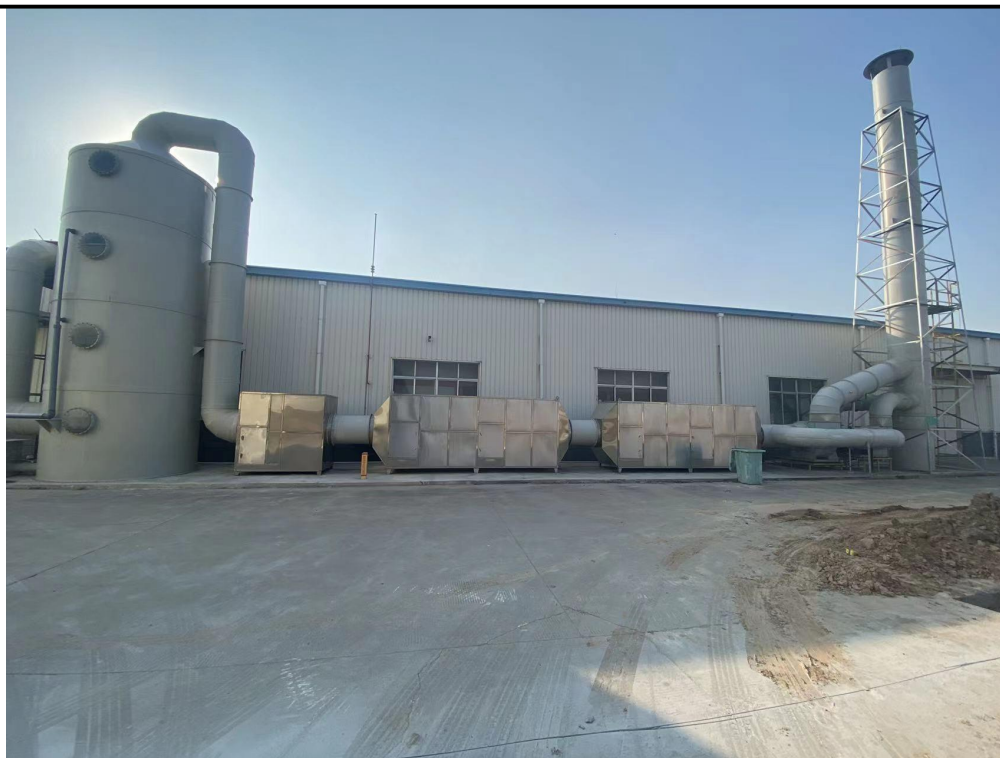
喷漆废气处理设施：喷淋塔+UV+二级活性炭，DA006
